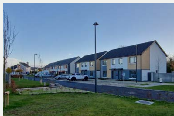
Boreen Bradach, Kinnegad 12-unit scheme, delivered by Westmeath County Council as part of the Accelerated Delivery Programme
